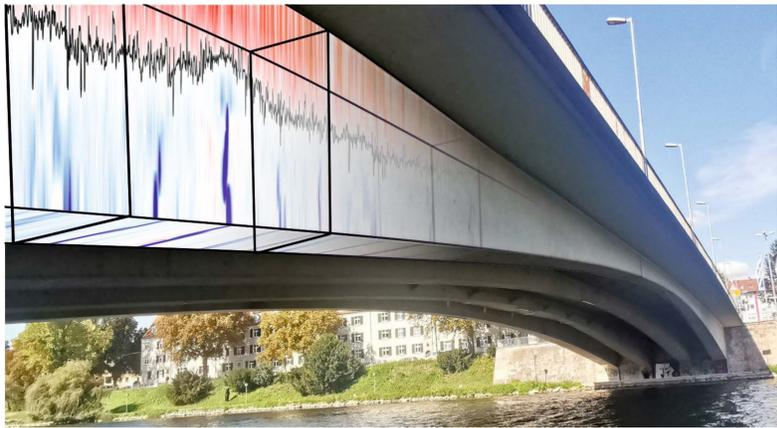
Figure 1: Transparent infrastructure; internal strains made visible by coda waves
